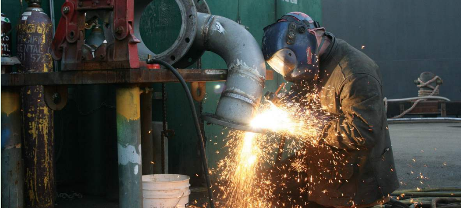
A welder is at work at Foss Shipyard in Seattle. Experienced craftsmen at the yard have expertise in all required skills in vessel maintenance and repair.
