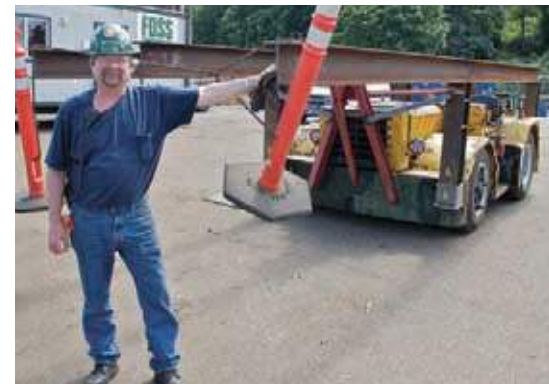
Gene Downie with framing he designed to simplify steel replacement in the barge's hull.
