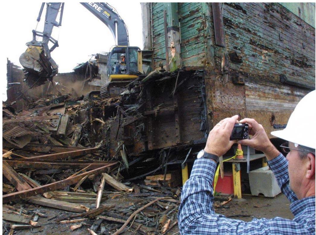
Project Manager Van Vorwerk shoots a photo as the month-long demolition process begins.
