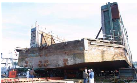
Level wooden runways were built at Foss Terminal to support the old drydock as it rolled slowly from the barge.
