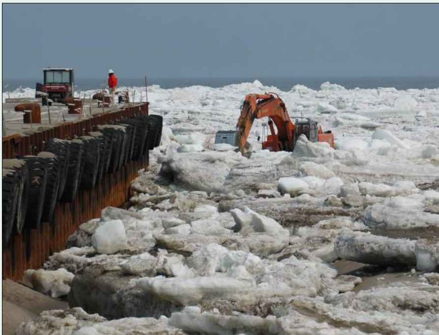
The Chayvo landing site was still icebound in late May. The Foss fleet finally got the green light to enter the port in early June.
