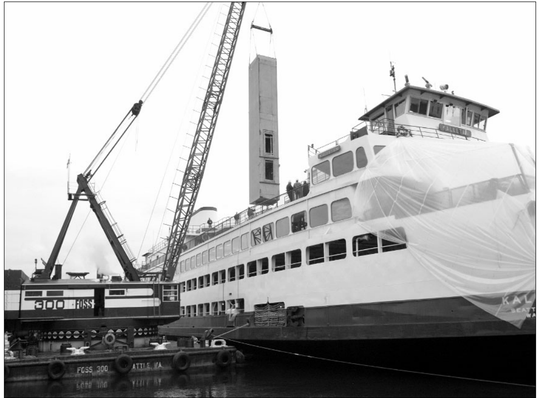
The steam derrick Foss 300 lowers a 47-foot-long, 33,000-pound elevator shaft into the Washington state ferry Kaleetan.
