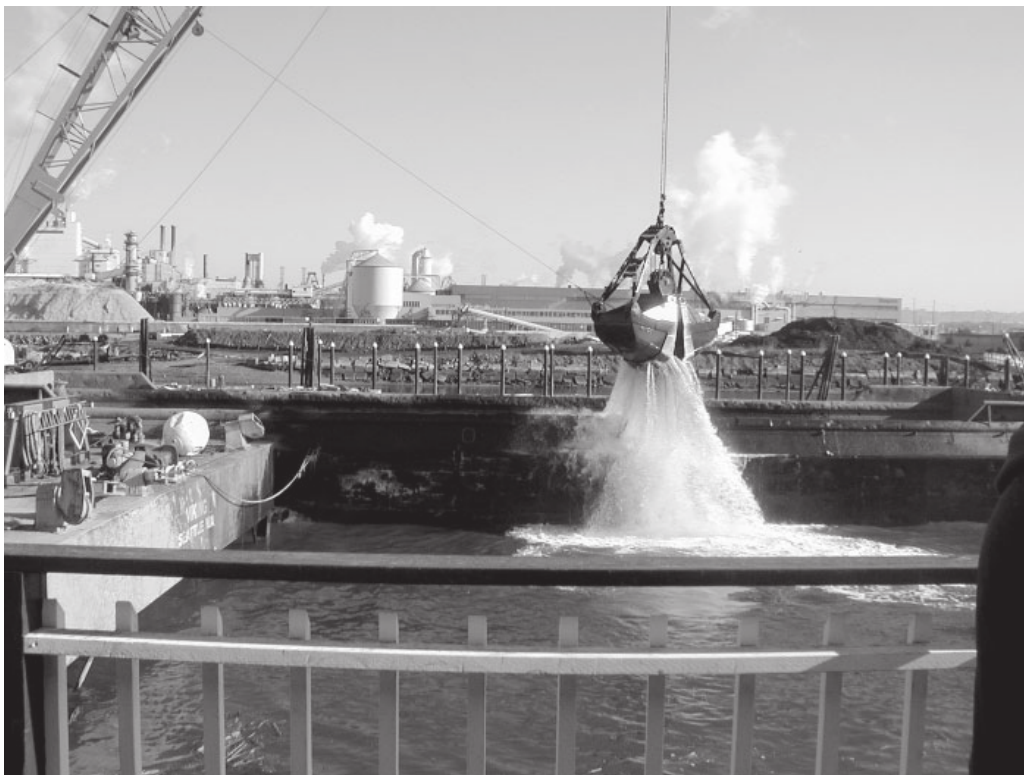
A clamshell dredge is at work in this photo taken from the porch of the Foss Tacoma office.
