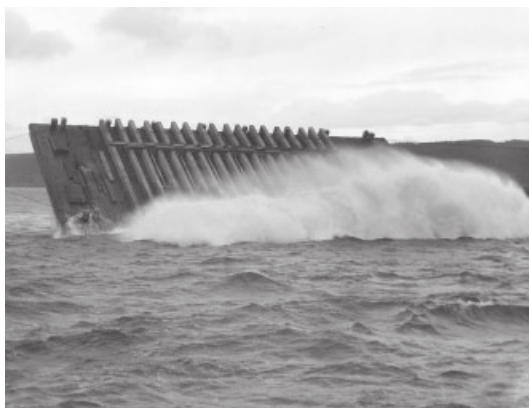
The concrete anchor has just slid off the barge into the Narrows. (1939)
