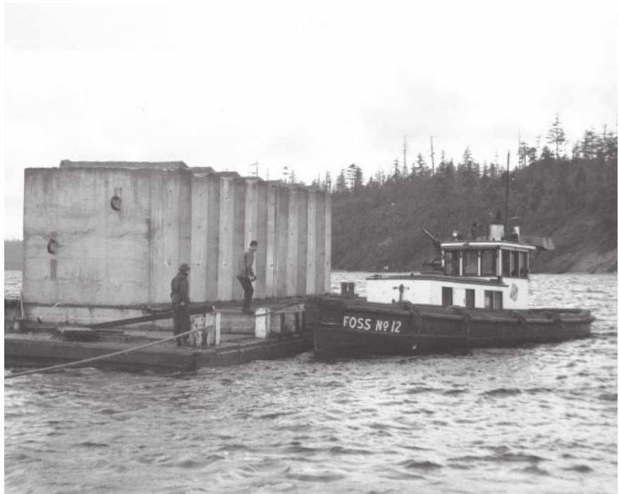
The crew of tug Foss No. 12 prepares to flood the port side of the deck barge to allow the 600-ton cement anchor to slide off into the appointed location in the Tacoma Narrows. (1939)
