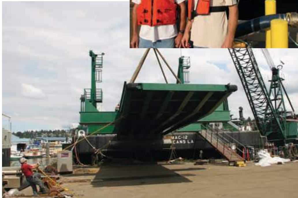
Jim Fox holds the tag line as the derrick Foss 300 lowers a new ramp into place on the barge Marmac 12 . The ramp measures 60-by-16 feet and weighs 44 tons.
