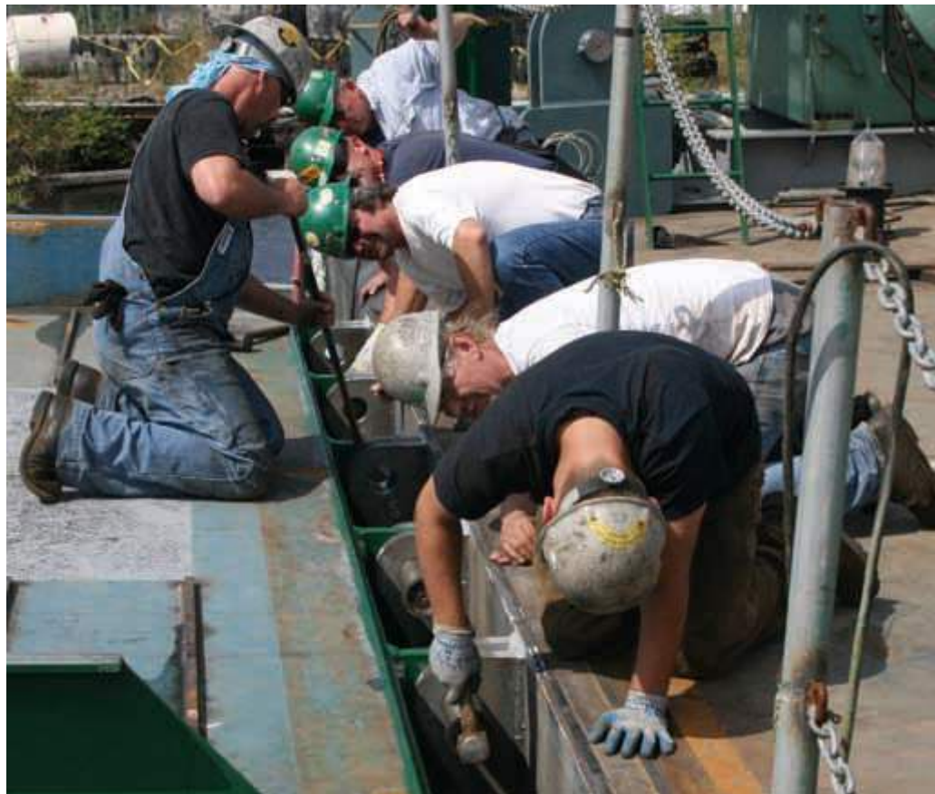
Johnny Warnes , left, uses a bar to align the ramp's hinges as Brandon Gipson , foreground, pounds in a pin. Behind Gipson are, from front, Joe Carl , Gene Downie , Steve Sorg , and Monte Roy .
