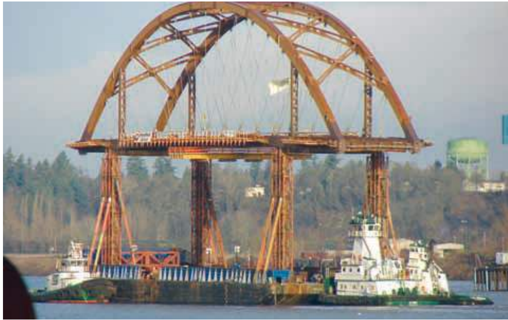
With good weather and smooth water, four Foss tugs move Portland's new Sauvie Island Bridge up the Multnomah Channel. The tugs, from left, are the Daniel Foss , PJ Brix and Jim Moore . The Betsy L is out of sight on the other side of the barge.
