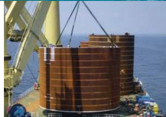
Deck-mounted cranes lift a 200-ton anchor, preparing to place it in about 300 feet of water.
