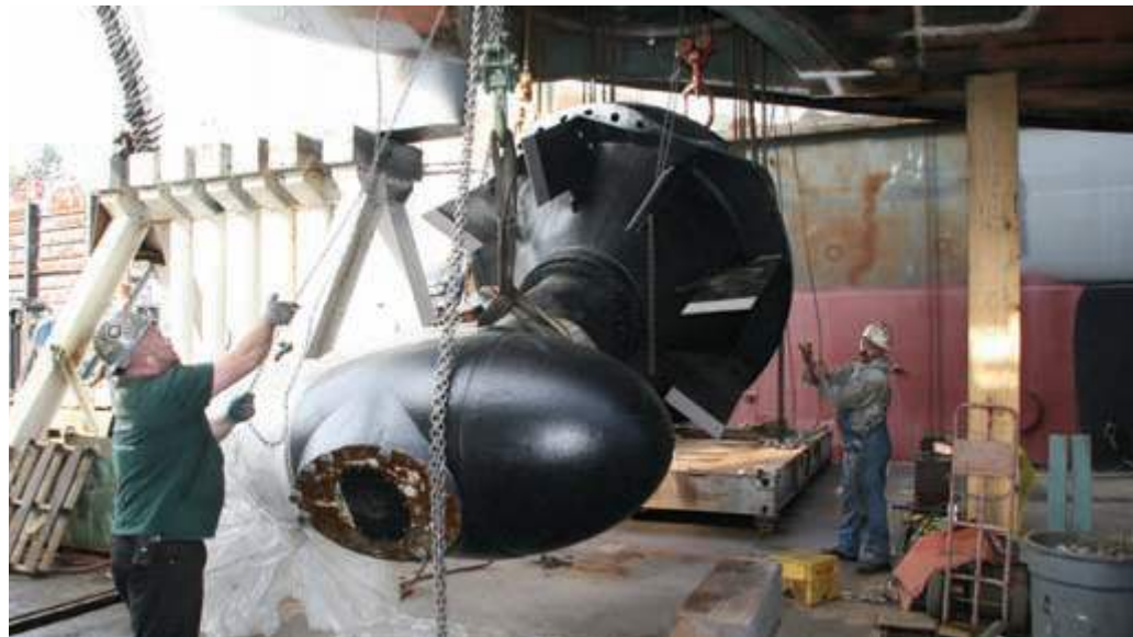
Terry Dawley, left, and Johnny Warnes hoist a new Z-drive into position on the Brynn Foss , the company's newest Tractor-Plus tug.
