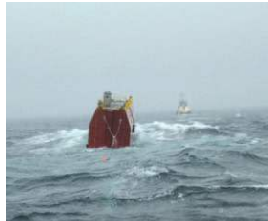
The caisson tips up in a wave during the trip from Portland up the coast of Washington.
