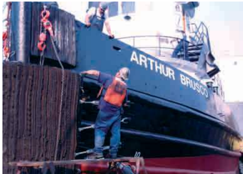
Rigger Terry Dawley , standing on the scaffolding, installs a new bow pud on the tug Arthur Brusco while Rigger Foreman Johnny Warnes observes from above. Partially visible under the scaffolding is rigger Damieon Dorosky . Welder Long Co is working on the pilothouse. Van Vorwerk Photo
