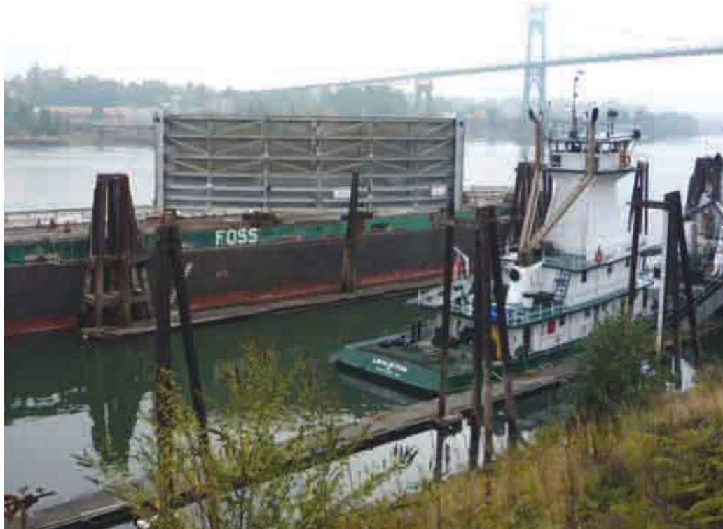
The lock gate sits on the barge Seattle in Portland, awaiting transport to the John Day Dam by the tug Lewiston , right.
