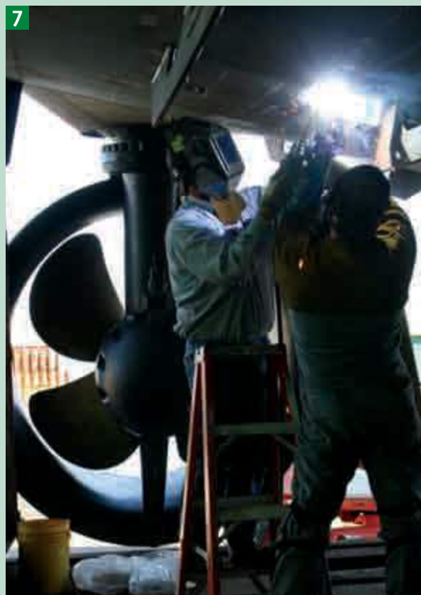
7 Welders work on the tug's bottom, with a newly installed Z drive in the background.
