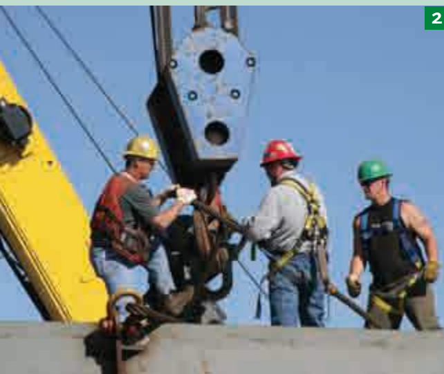
2 Rainier workers adjust the rigging on the stern section before it is lifted for its short upriver voyage.
