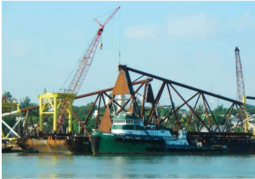
The Lauren Foss and its barge are moored at the Commsa fabrication yard in Tampico, Mexico. On the barge is a 237-metric-ton pipe assembly called a “tripod jacket,” which is a support leg that will rest on the sea floor as part of the offshore platform's structure.
