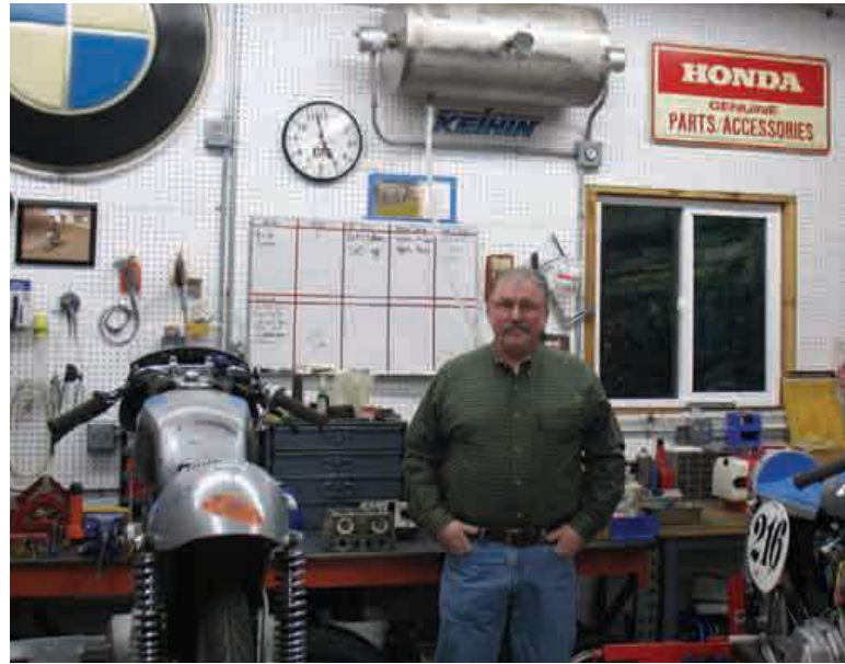
Mark Troutman built the hybrid system that heats his shop. Above his head is the storage tank for the heated water that circulates through the floor.
