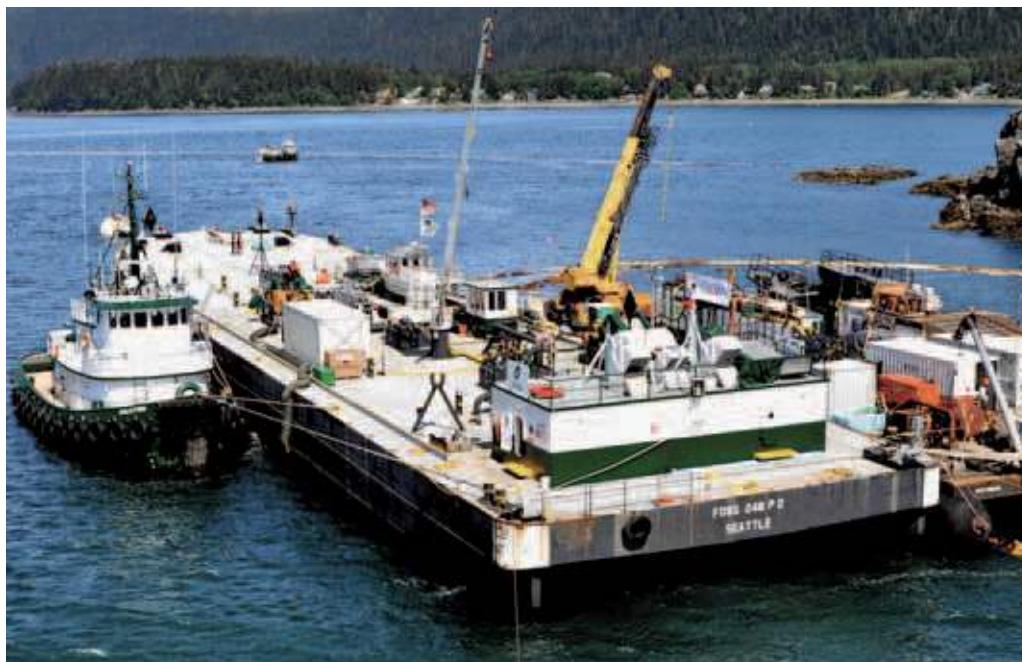
The Halle Foss and the tankbarge 248 P-2 on the job over the wreck of the Princess Kathleen .
