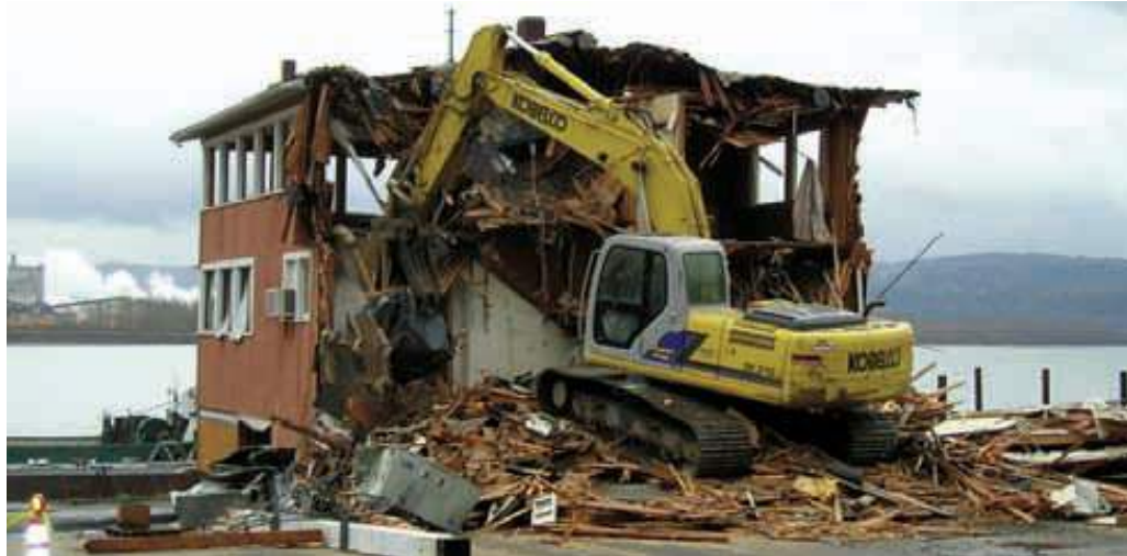
An excavator spent about an hour chomping through the old office building at Foss Rainier Shipyard on Wednesday, March 26.
