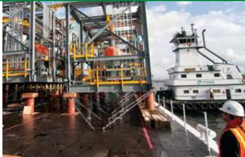
Project Manager Steve Gormiak of Foss watches as a module is loaded onto a Foss Barge at the Port of Vancouver.
