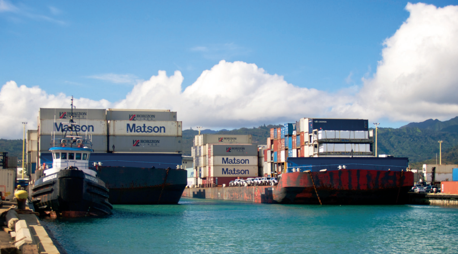
The Tug Manuokekai and two of Young Brothers' four new barges, berthed at the Port of Honolulu.
