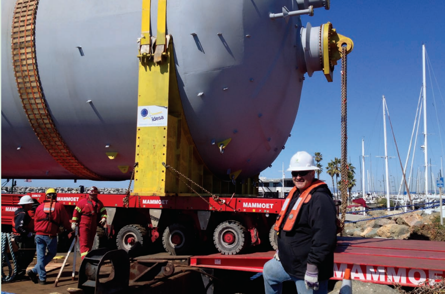
Southern California Port Capt. Paul Hendriks supervised the coke drum project for Foss. Behind him, one of the drums is moved over a ramp from the barge ZB 240.
