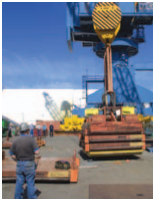
Rigger Foreman Jim Mosman , foreground, looks on as one of the cranes is tested with a 160,000-pound weight.
