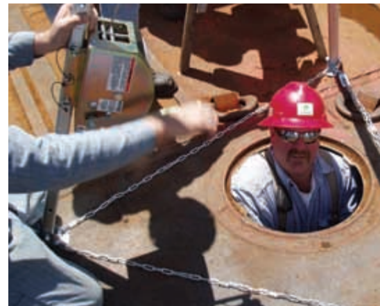
Todd Hall of Foss Rainier Shipyard descends into a ballast tank on the barge BMC 6 during the confined-space rescue drill.
