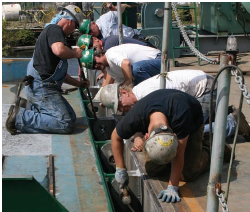
Johnny Warnes , left, uses a bar to align the ramp's hinges as Brandon Gipson , foreground, pounds in a pin. Behind Gipson are, from front, Joe Carl , Gene Downie , Steve Sorg , and Monte Roy .
