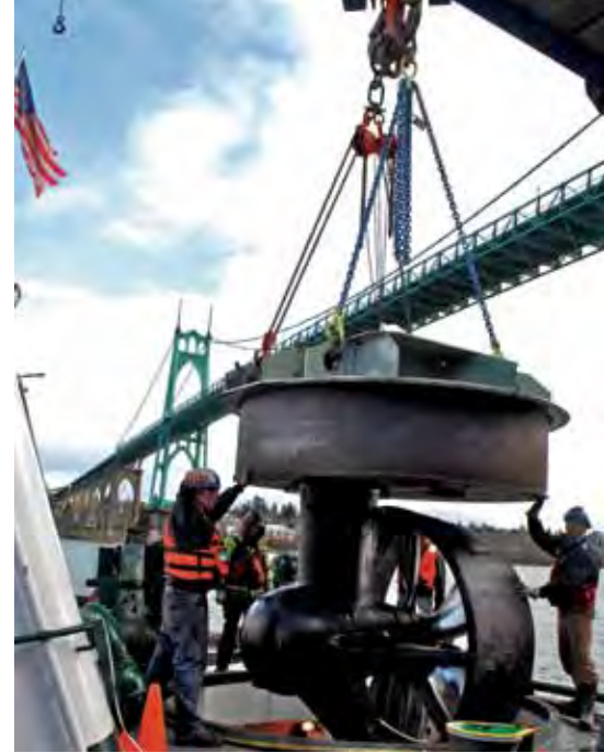
Workers at Advanced American Construction install a rebuilt Z-Drive in the tug PJ Brix . The tug remained in the water for the job.
