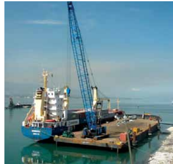
The Foss barge Columbia Boston was set up by ACTC as a temporary cargo terminal in Port au Prince
