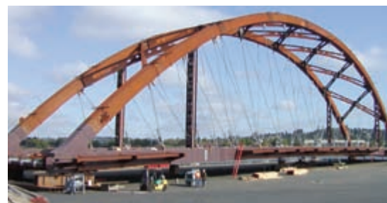
The Sauvie Island Bridge span at Terminal 2 in Portland, ready to be moved by Foss
