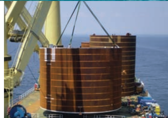
Deck-mounted cranes lift a 200-ton anchor, preparing to place it in about 300 feet of water.
