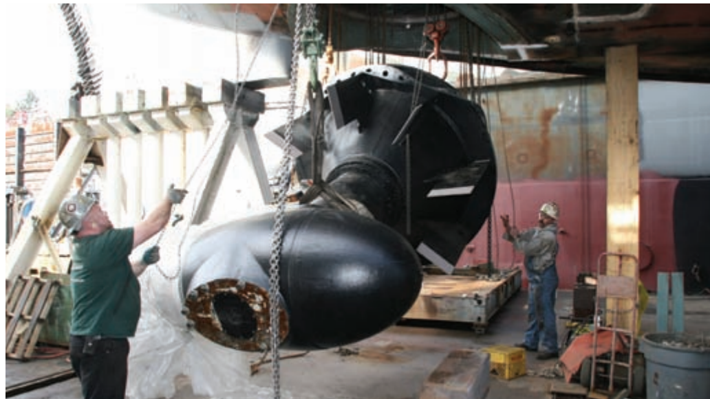
Terry Dawley, left, and Johnny Warnes hoist a new Z-drive into position on the Brynn Foss , the company's newest Tractor-Plus tug.
