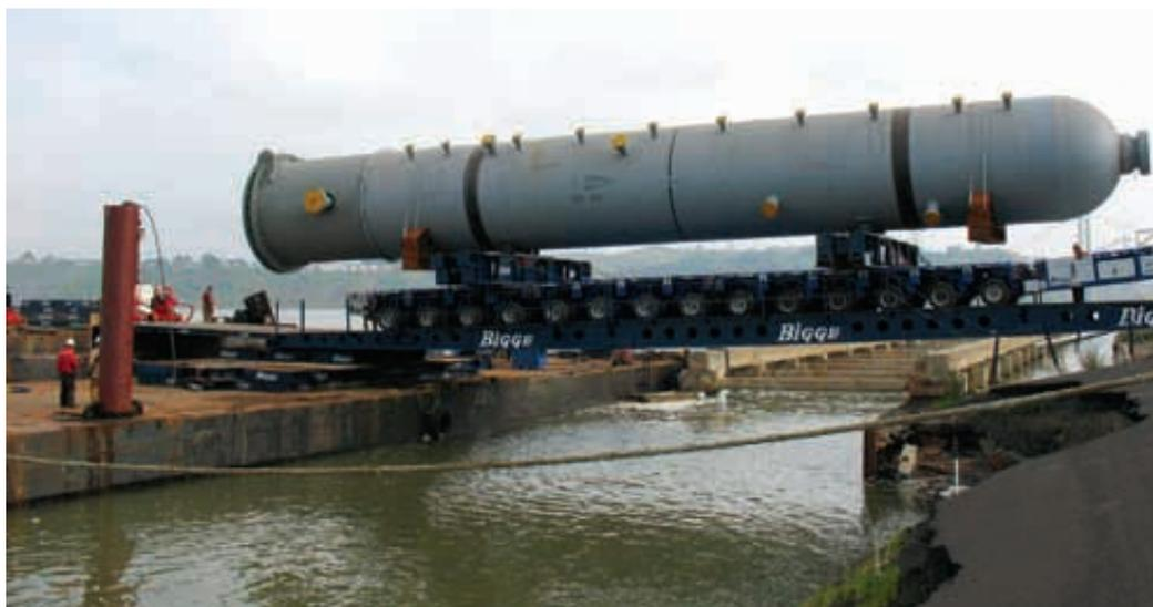
One of three hydrocrackers rolls over a ramp from a spud barge to the ConocoPhillips’ refinery.
